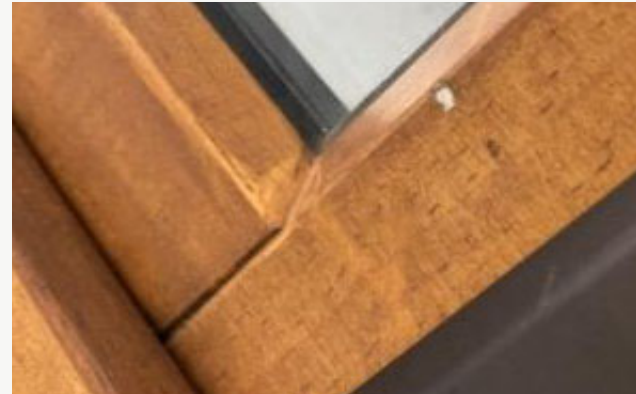
No coating degradation visible after 14 years
