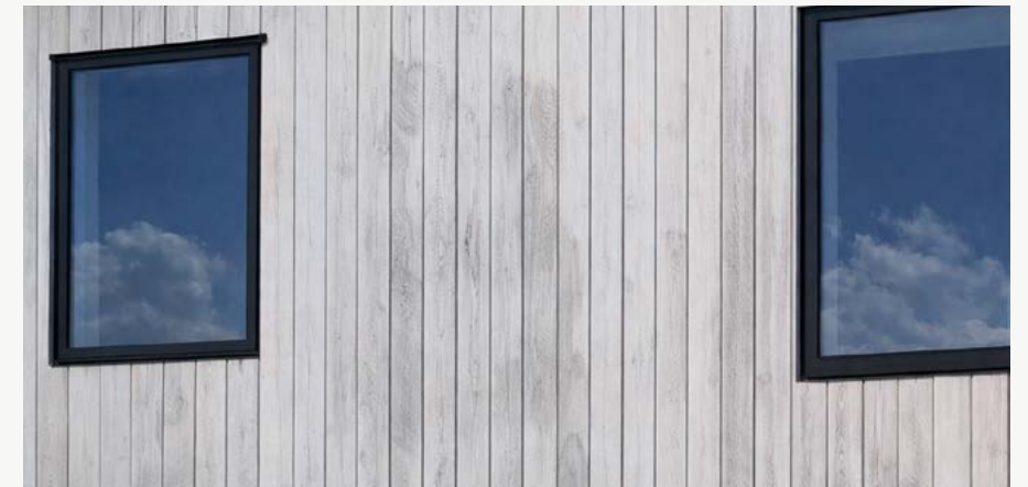
A New Zealand housing project with a distinct batten (sub-frame) silhouette, showing on the cladding surface
